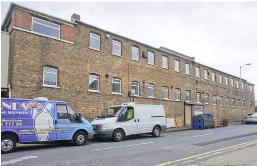
Tileyard Road (front) elevation
