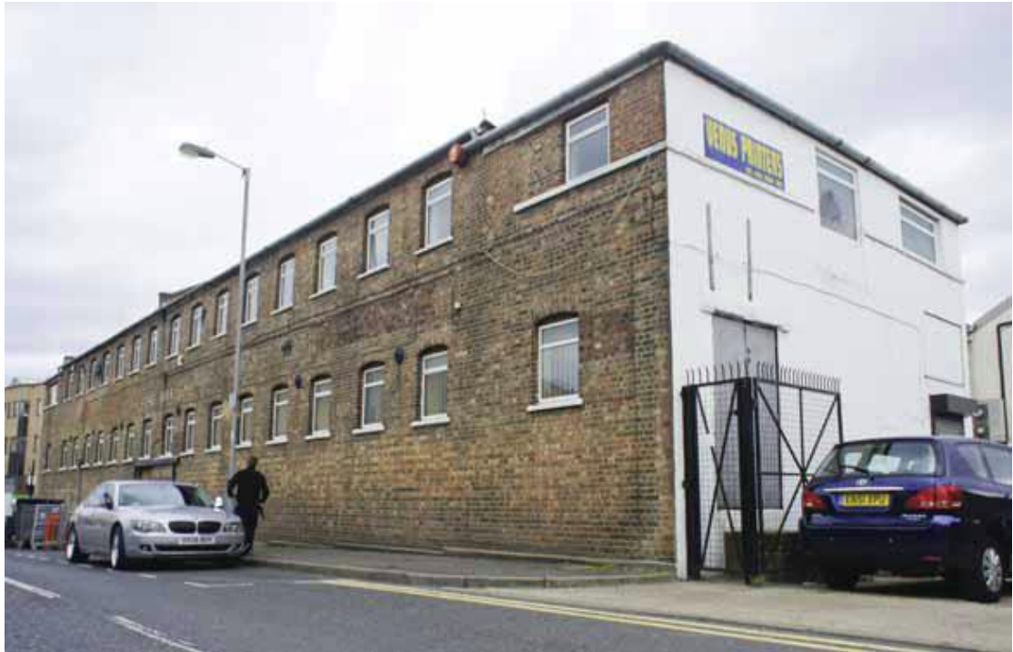
View along Tileyard Road, with the existing service bay to the right. York Way sits to the far right of site the right.
